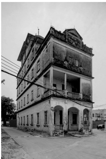
A 5-storey school financed by the owners of The Sun Department Store 大新公司 in 1930 (Author in Wai Sha village 外沙, Tang Jia Wan 唐家灣, December 2017)
