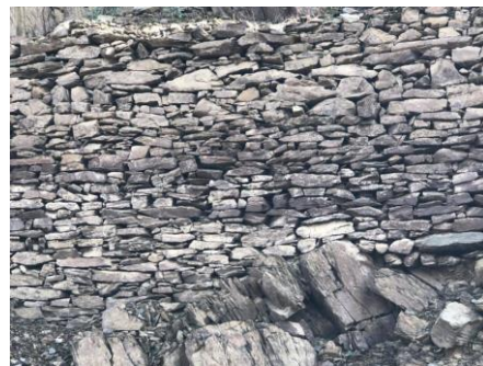
Close-up of stonework supporting the water race Photo: Kira Brown
