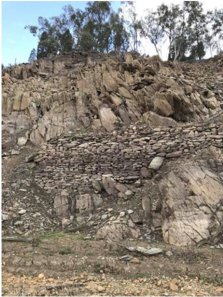
Part of the stonework supporting the water race which is fully submerged when the dam is full Photo: Gilian Oxley
