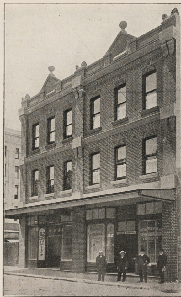
The original Edwardian shop fronts at 82-84 Dixon Street.
